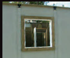
Windows & Blast Panels
