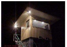
The Tower roof has a 3 foot over hang on all sides. It has three windows; two windows on each side and a larger window on the front. The side windows measure 3' x 3' while the front window measures 8.5'x 3'.
